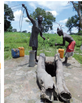
South Sudan 2016/17/18: Repair and construction of water wells with hand pumps
